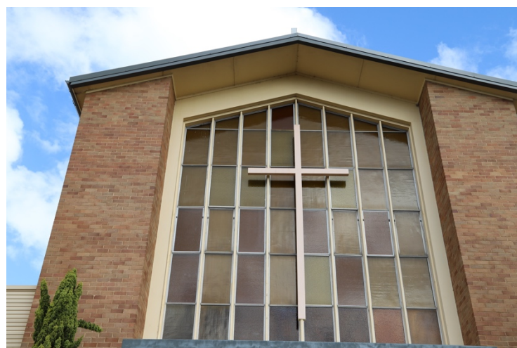
AFTER: Timber barge capping on the front of the church has been replaced with Colourbond and eleven glass panels have been replaced.
