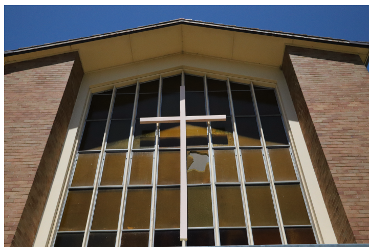
BEFORE: Timber barge capping on the front of the church has degraded, glass panels are broken and cracked.
